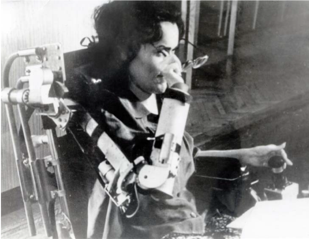
Figure 2.4: One of the first active arm orthoses powered by electromagnetic actuators, developed at the Mihailo Pupin Institute, being controlled with a joystick by an individual suffering from a muscular dystrophy (reproduced with permission from Stanic (2018)).
