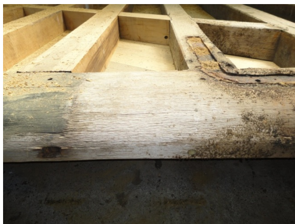
Figure 24: Deteriorated wood at the water line of an Oak door. Note that the door is being renovated and some parts are already replaced.
