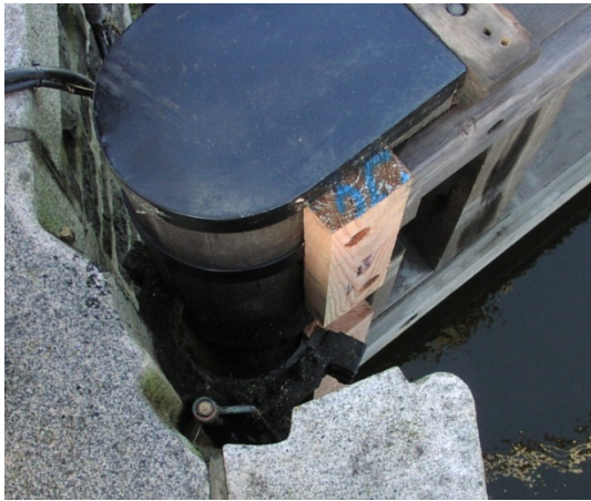
Figure 22: Quoin post and door during hanging in the door. (Wijma Kampen B.V. (2012a))
