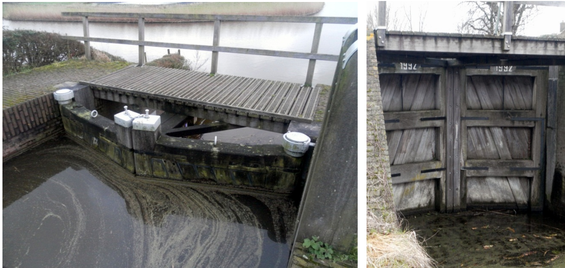
Figure 43: Wooden mitre gate under water level difference loading
