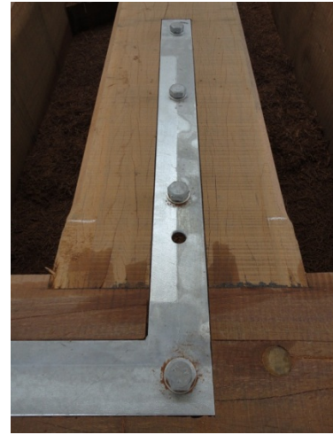
Figure 18: Tight fitting of the connection
