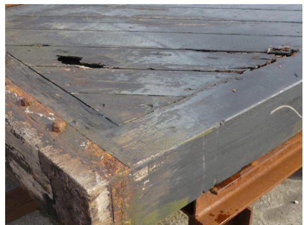
Figure 25: Deteriorated planking of an Oak door (Van Dongen, 2012)
