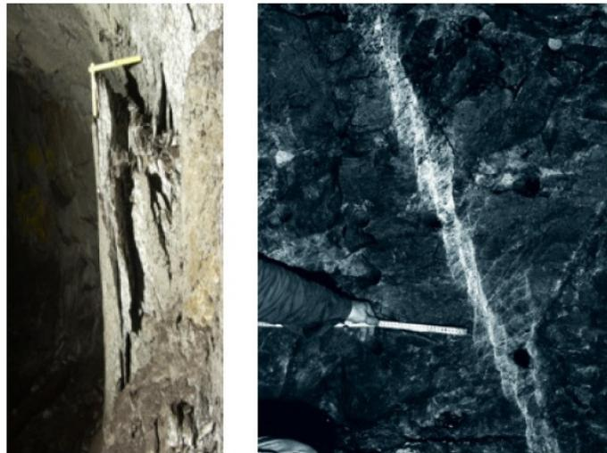
Figure 58: Spalling at unconfined tunnel walls and shear failure in confined zones. (Kaiser, *et al.*, 2010)
