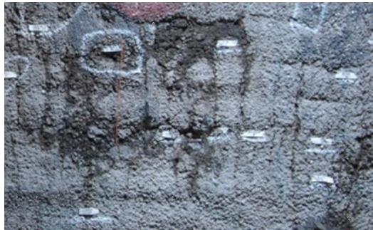
Figure 6. Location of reinforcement bars visible in Panel 2
