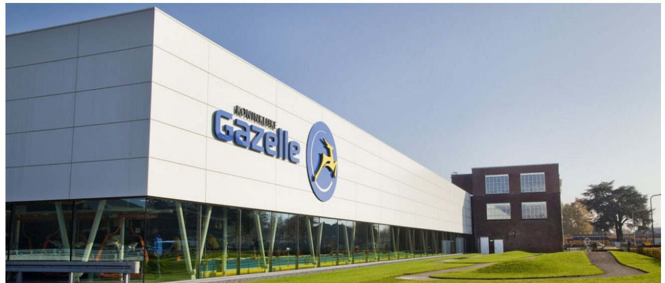
Figure 1 Gazelle and Union factory and office in Dieren
