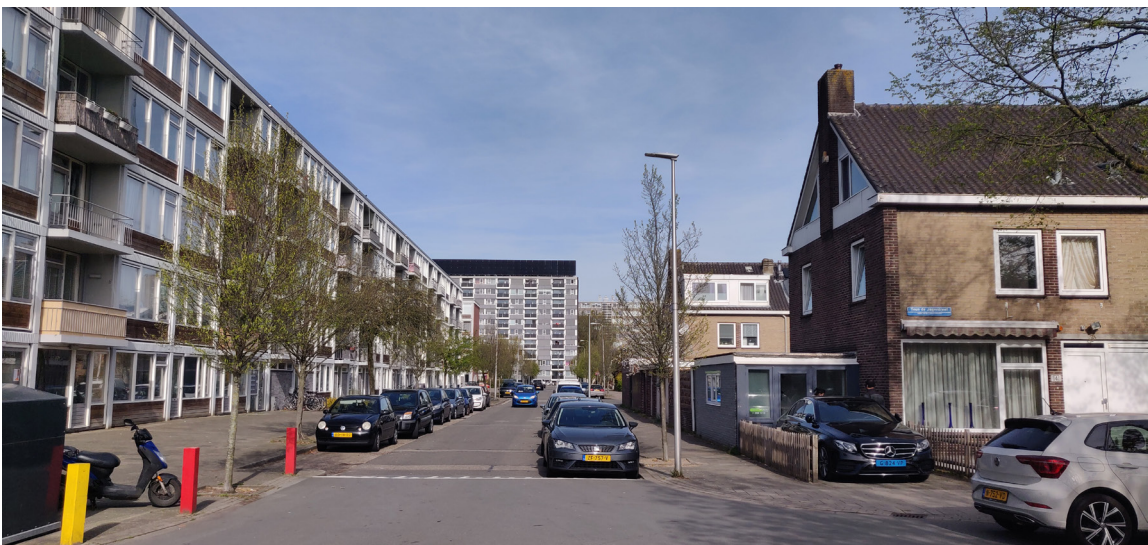
Figure 20: Perspective taken from the Ebrodreef. The building on the left shows a transformation of the ground floor. From storage space to living space. This creates "eyes on the street". It shows awareness of the shortcomings of the original architecture. Date: 04/2022
