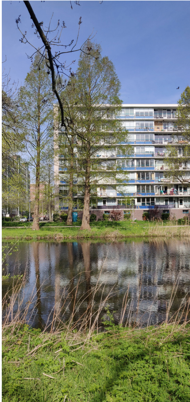
Figure 23: Perspective from the Marnedreef facing a high rise building alongside the Watertorenpark. It shows the attention to green space after the intervention in 2005 where waterfronts were dense and diversified. Date: 04/2022
