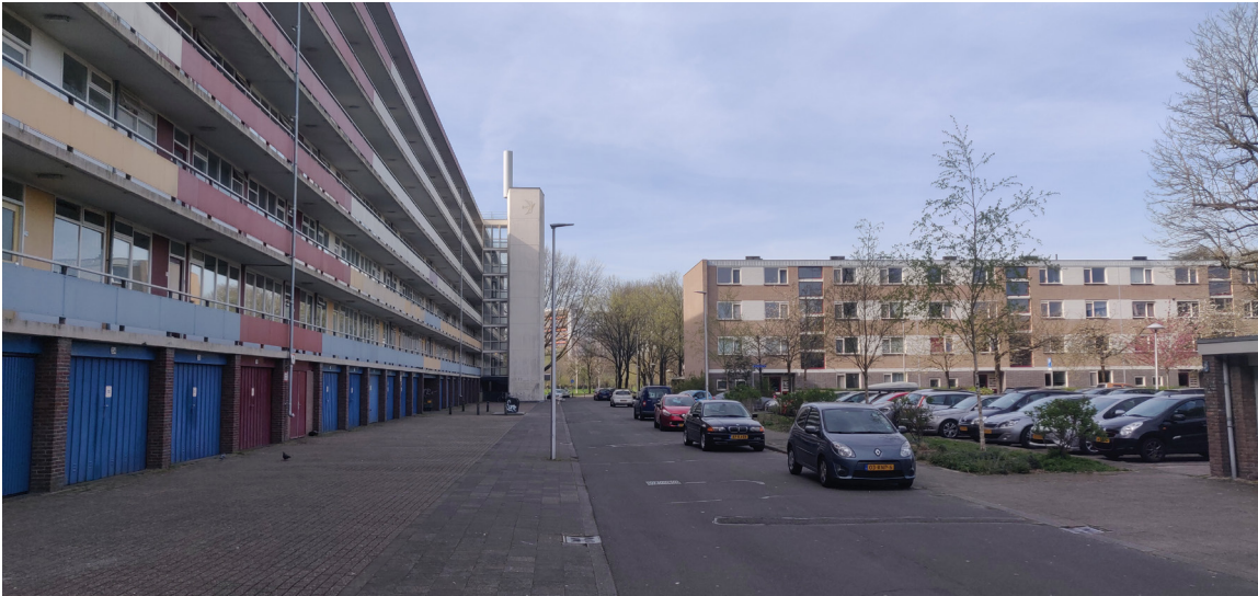
Figure 18: View facing the green structure of the Oberondreef. This image shows the troubling architecture of the plinth. Contrasting to the green structure this part has a lot of paved surface. The anonymous feeling is amplified by the cold meeting of the storage spaces at the ground floor. Date: 04/2022
