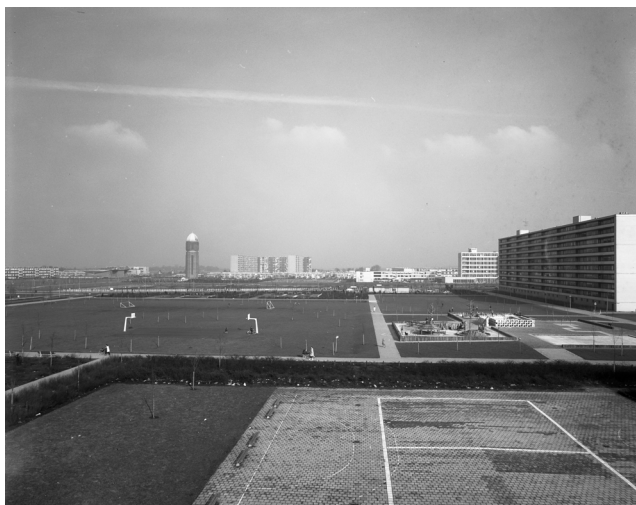
Figure 4: View towards the playground on 'La Bohèmedreef' in Utrecht; on the right the highrise building along the 'Faustdreef' and in the background the Overvecht watertoren. Date: 1971 / Collectie Het Utrechts Archief [805298]
