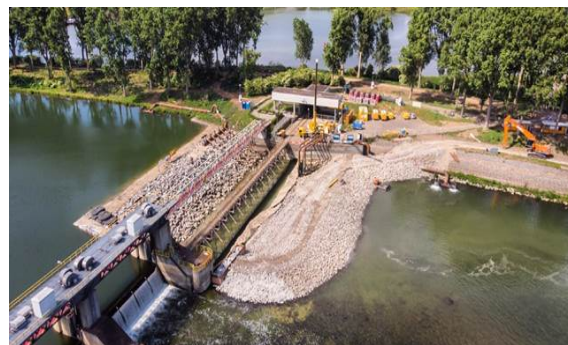
Figure 2.13: reparation of weir Linne [52]
