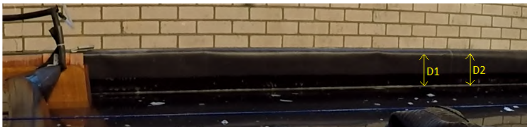
Figure 6.15: water depth measurement
