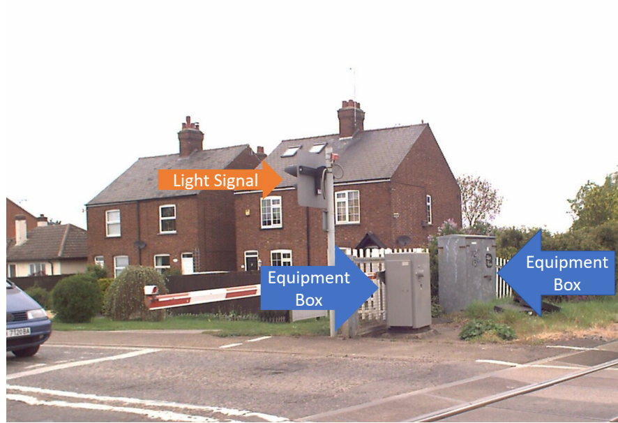
Figure 4.4: Cross road in the railway near Ely, UK. The illustrated equipment boxes are different than the boxes used for training. As a consequence, 2D detector was not able to capture them.
