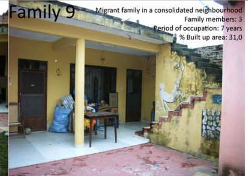
The first construction with 3 rooms and a kitchen a stair already leads to a future second floor
