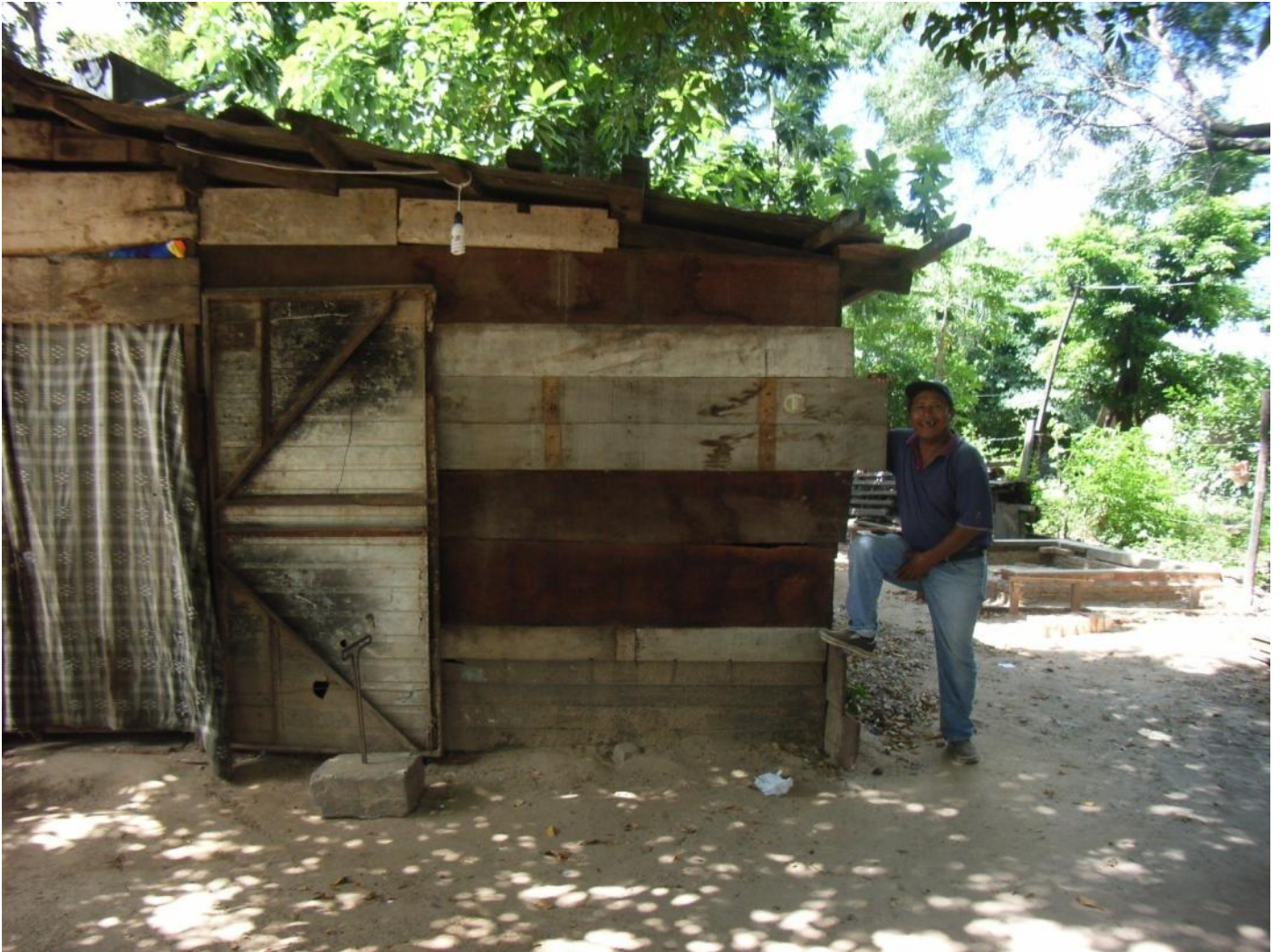
Fig. 4.12 Self constructed wooden house in Santa Cruz de la Sierra
