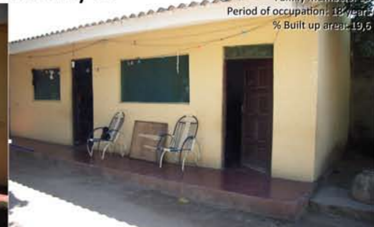
The first two constructions made with bricks and steel plates. They are used as bed rooms.
