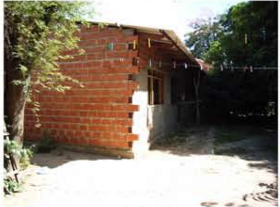
The newest construction for the son of the owner.
