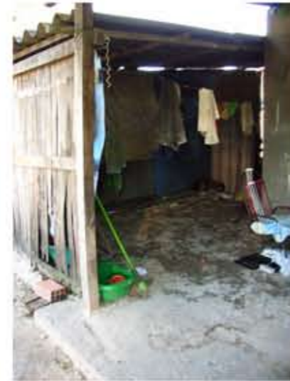
The temporary construction made of wood, metalsheets and plastic. These materials once served as materials for the family's first construction.
