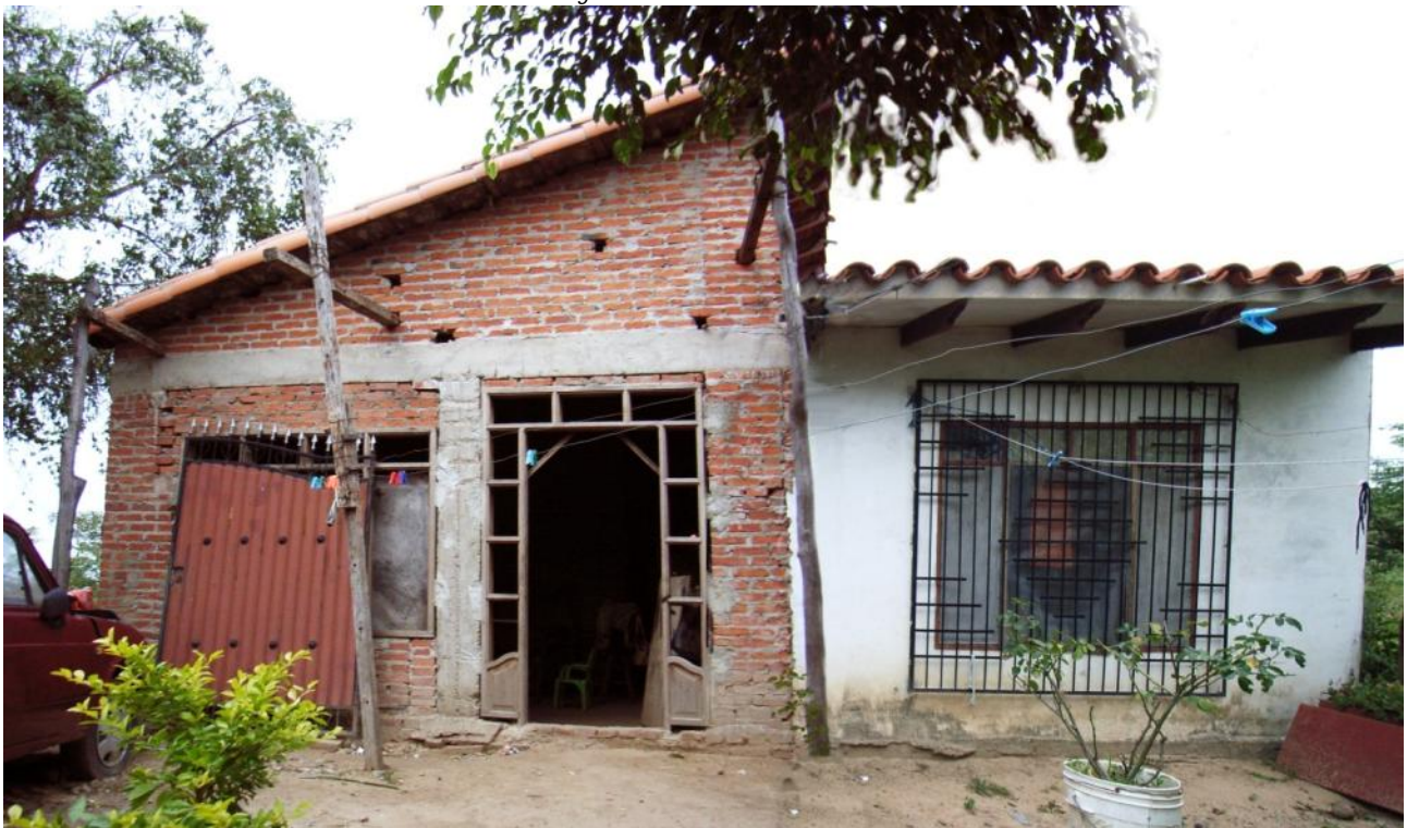
Fig. 3.17 constructed brick house in Santa Cruz de la Sierra.
