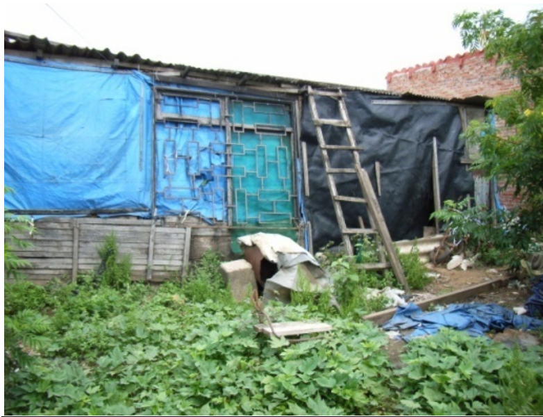
Fig. 3.15 Construction with loam, sheets of corrugated iron and plastic cloths
