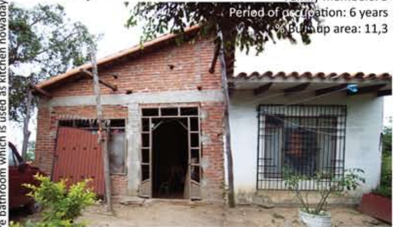
The white structure is the first construction, which was made directly with bricks and tiles and has a multifunctional usage.
