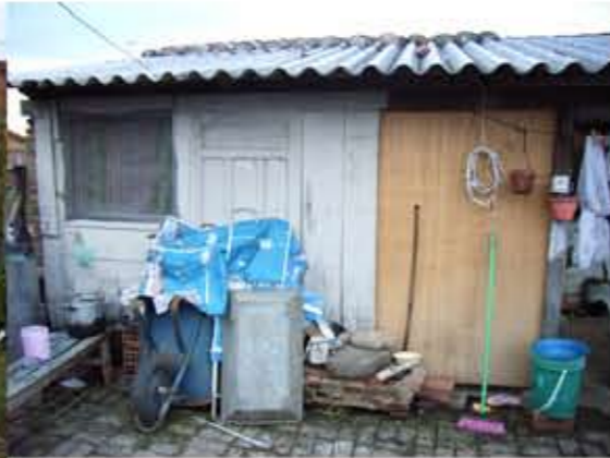
The facade of the kitchen
