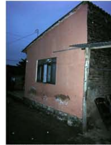
The first construction with 2 rooms
