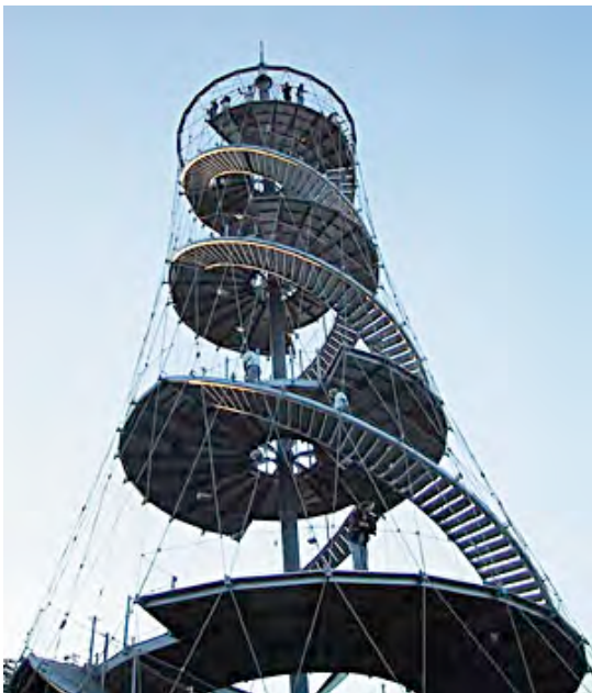
Figure 247: Killesberg tower, Jörg Schlaich, Rudolf Bergemann, 40 meter high. The tensile net structure provides a lot transparency, and a light weight structure.
