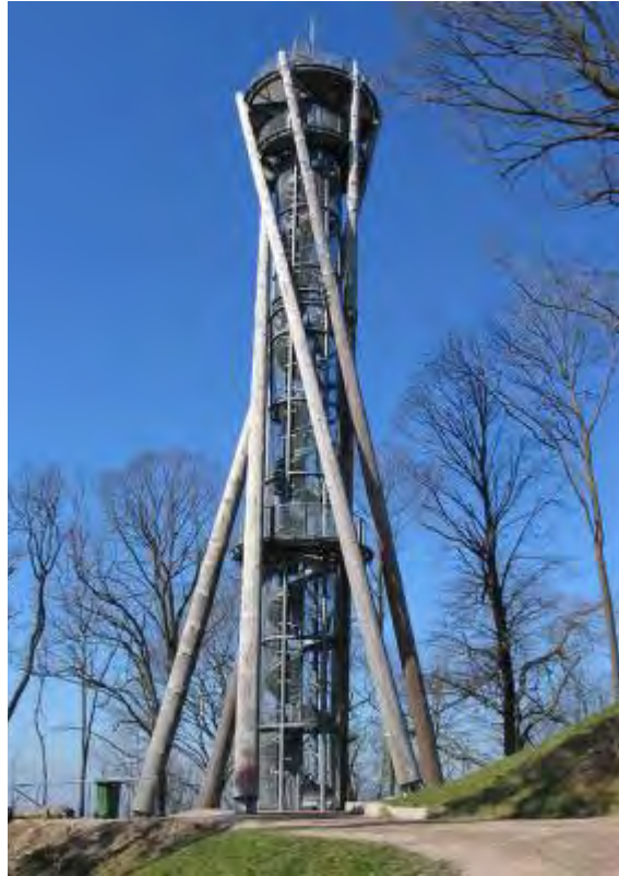
Figure 249: Observatory tower Schossberg, spiral staircase in between columns
