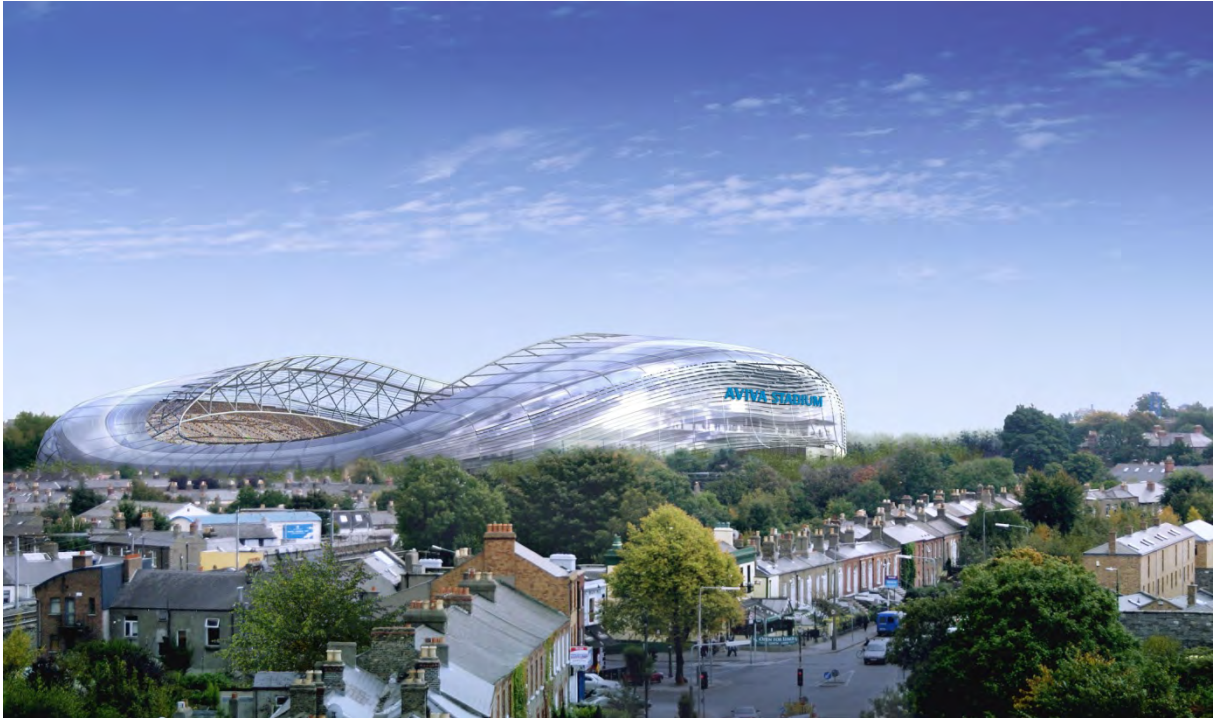
Figure 236: Polycarbonate sheet roofing, Aviaiv stadium, Dublin - realised
