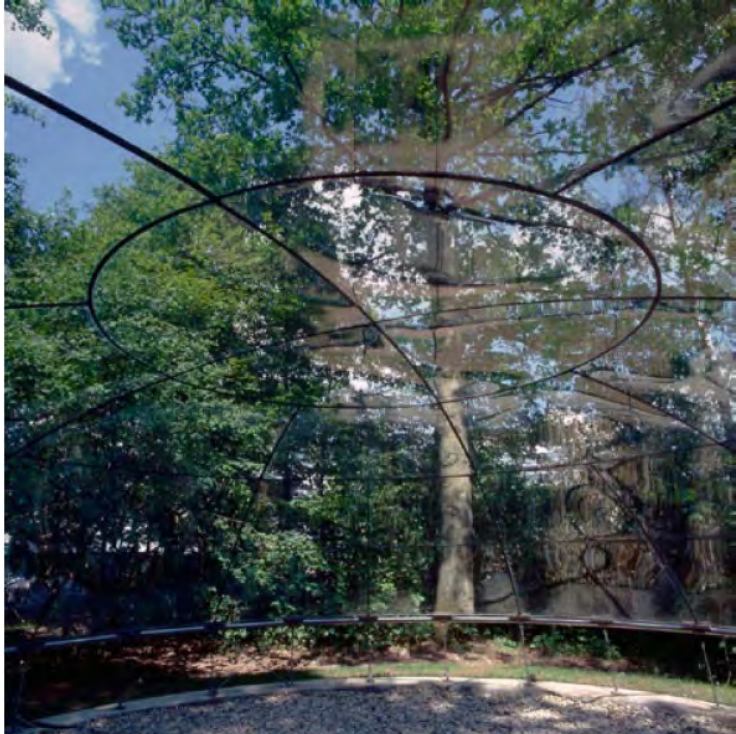
Figure 242: Glass shell without supporting substructure, Blandini & Sobek
