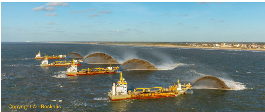
Fig. 2. Photo shows an example of nourishments of the coastal profile feeding the offshore sediment budget (photo courtesy of Boskalis).
