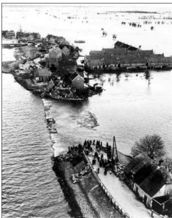
Figure 4.2: One of the hundreds of breaches in the Dutch dikes in 1953 (Source: ANP, library KNMI)
