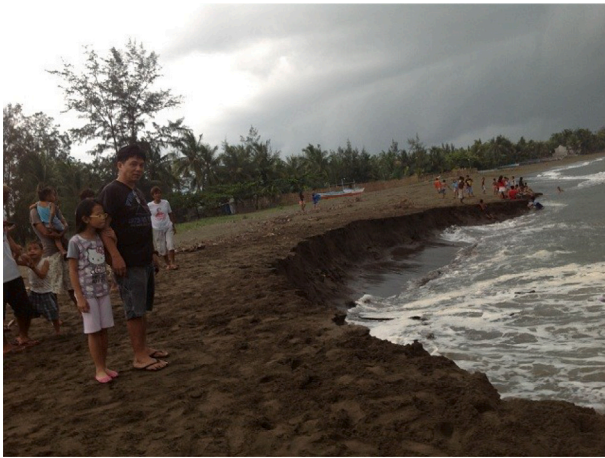
Fig. 7. Beach collapse in Candelaria- Zambales, Philippines, 2013 (photo courtesy of Mines and Geosciences Bureau, Manila).
