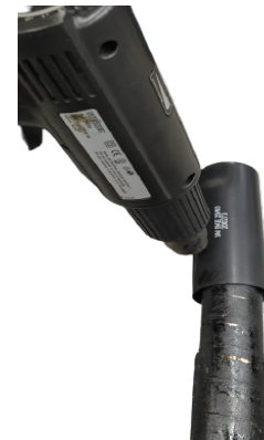
Figure 4.12: Fitting of Heat Shrink Caps
