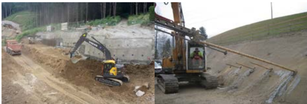
a) Standard soil nailing system
