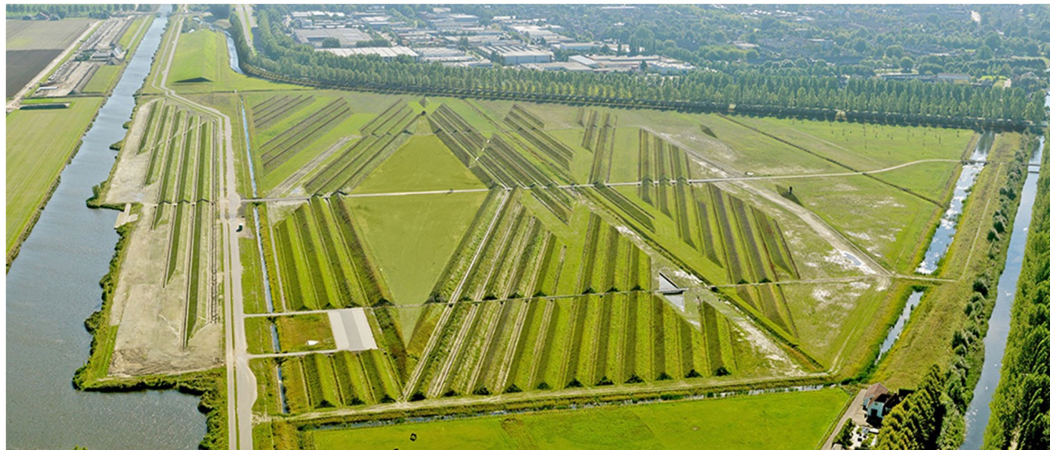
FIGURE 6 The Buitenschot Land Art Park is a recreational park with noise-reducing features, which reduces noise from airplanes and also provides the area with space for events and recreational areas.
