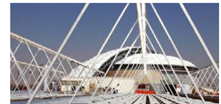
22.01 The solar installation of the stadium
