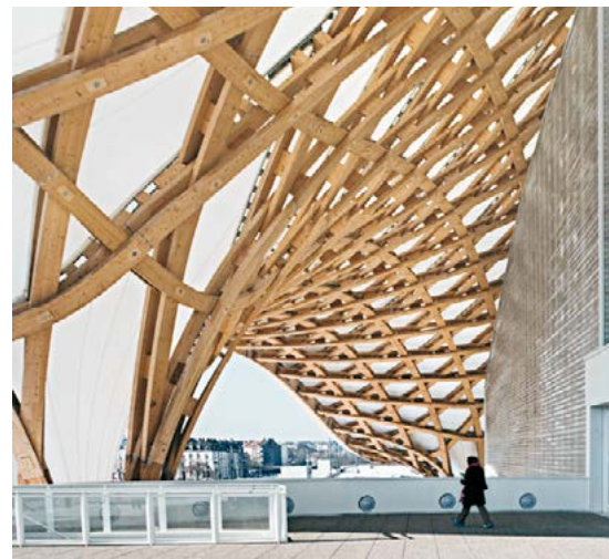
20.03 The wooden roof construction
