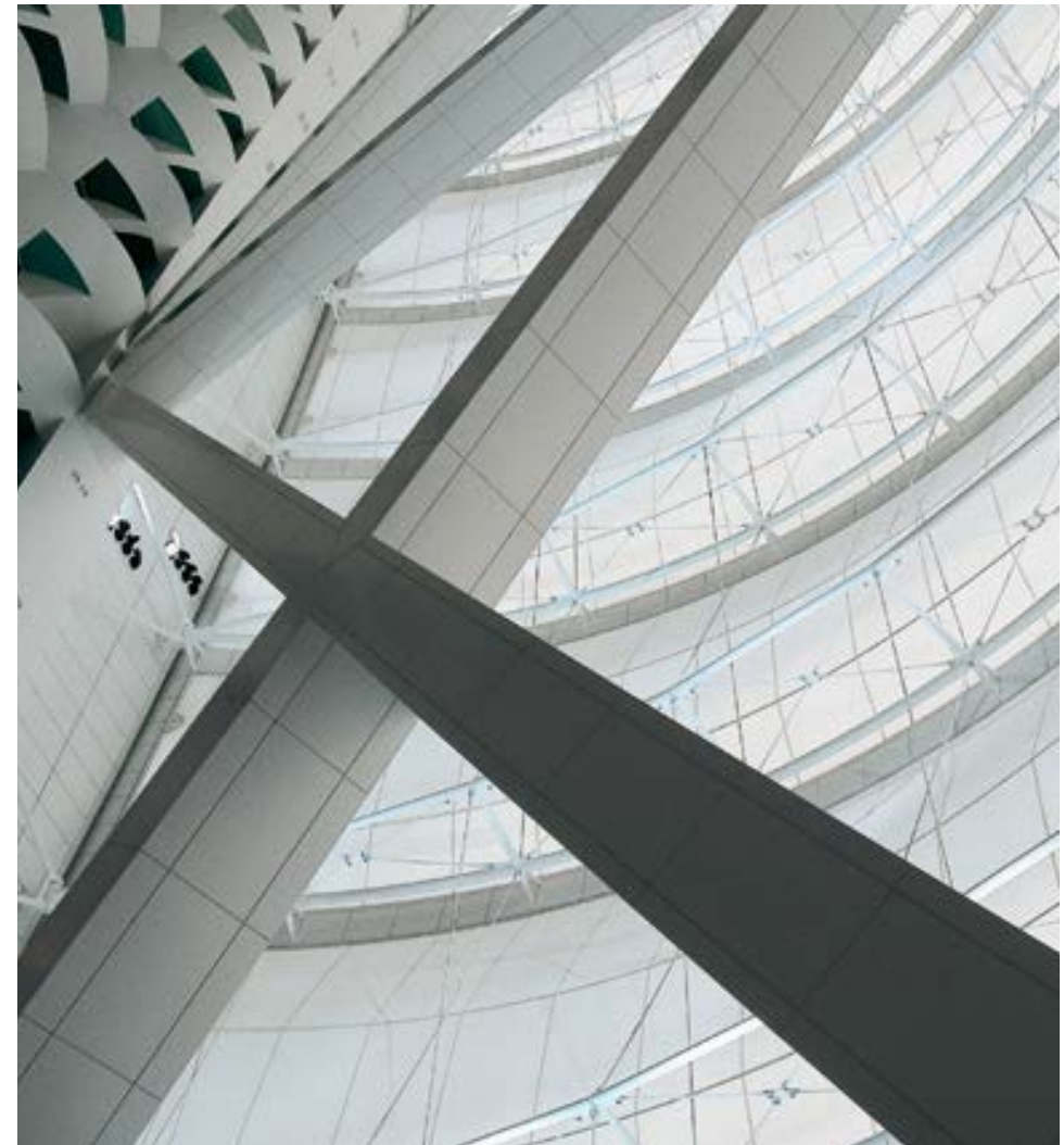
2.04 Atrium from ground level, giving a sense of the light conditions
