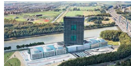
6.01 Overview of the Westraven building
