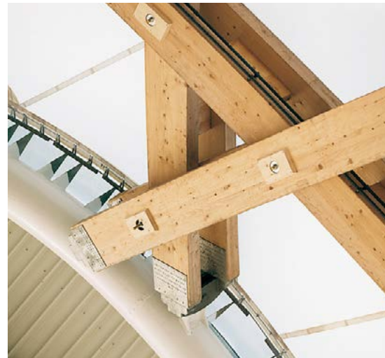
20.02 Detail of the wooden beams on the steel construction
