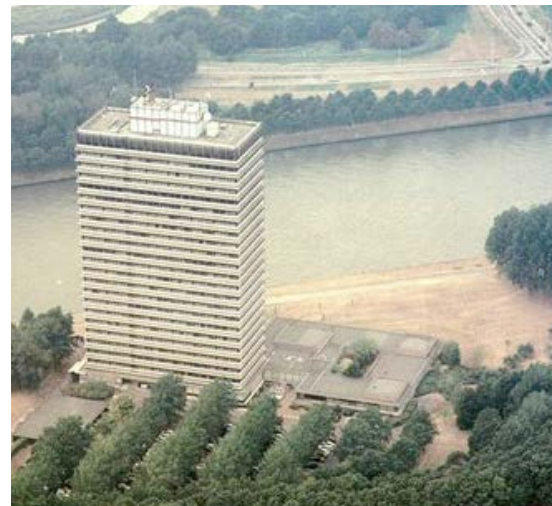
6.03 The westraven before the renovation
