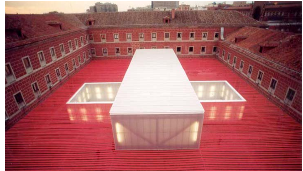
17.04 The pavilion from above, looking into the white spaces inside the container
