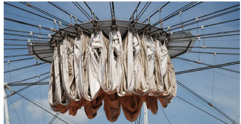
23.05 The roof is folded
