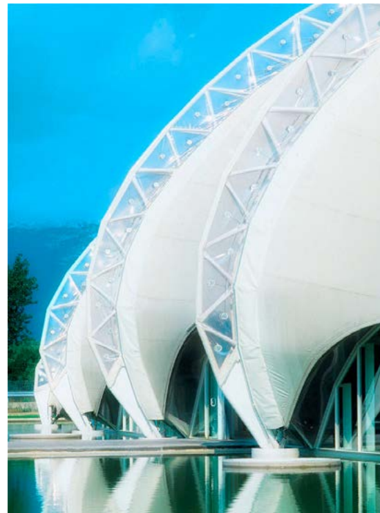
29.02 The roof connection to the ground
