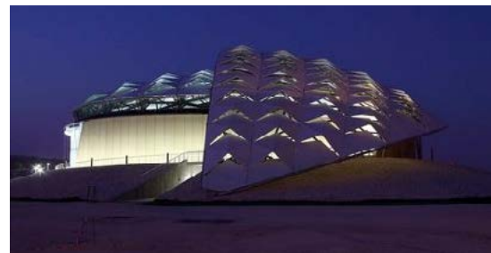
22.03 Roof openings are seen at night
