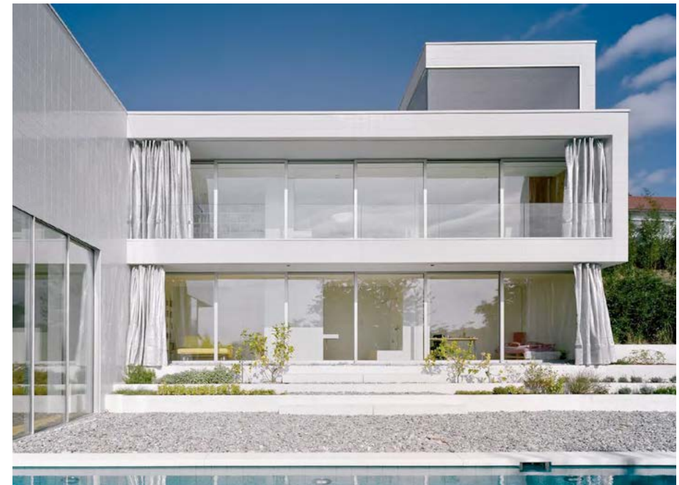
4.04 The façade with open curtains
