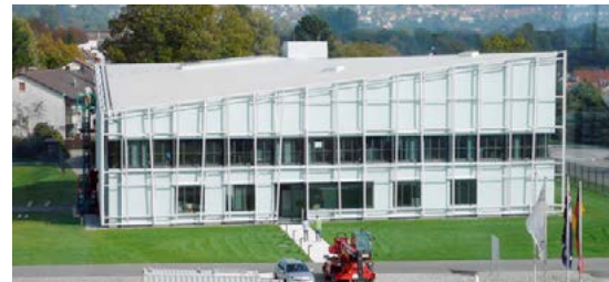
5.03 Inner façade is showing during construction
