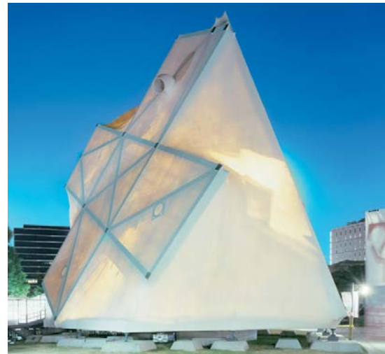
30.02 Illuminating Prada Transformer
