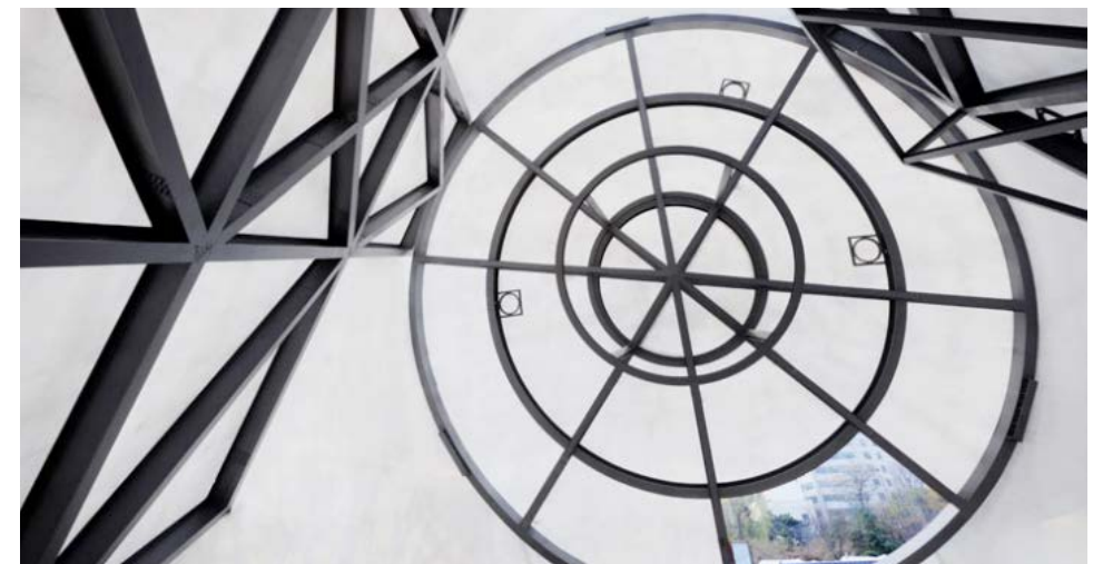
30.05 The construction inside the Transformer
