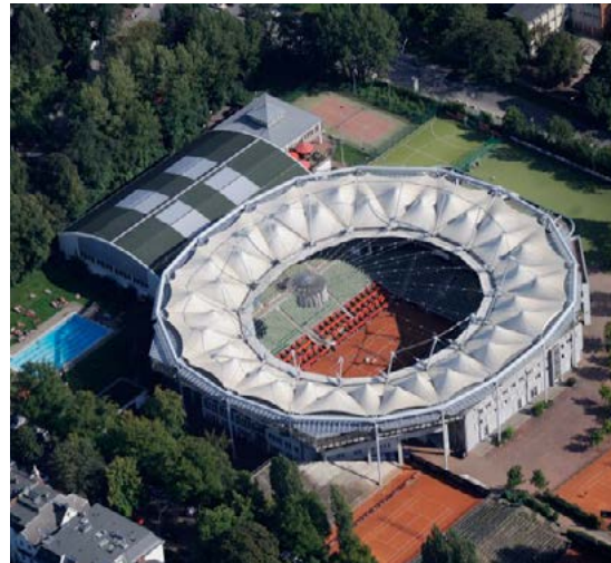
23.02 Bird's eye view on the tennis court with open roof
