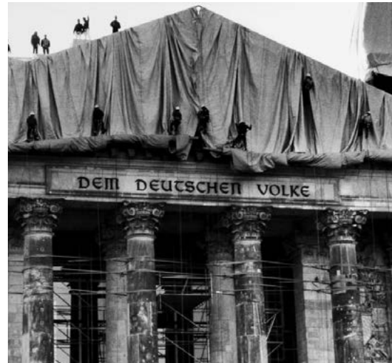
7.02 Workers wrapping the Reichstag
