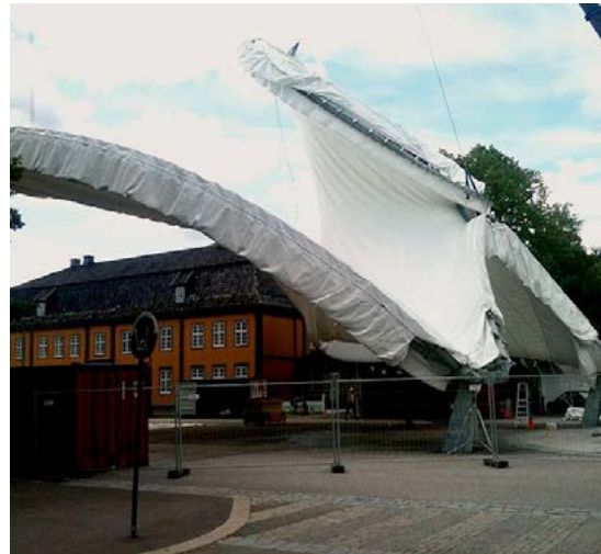
35.02 The installation of the Tubaloon
