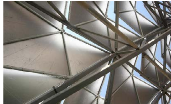
22.02 Inside of the roof cladding
