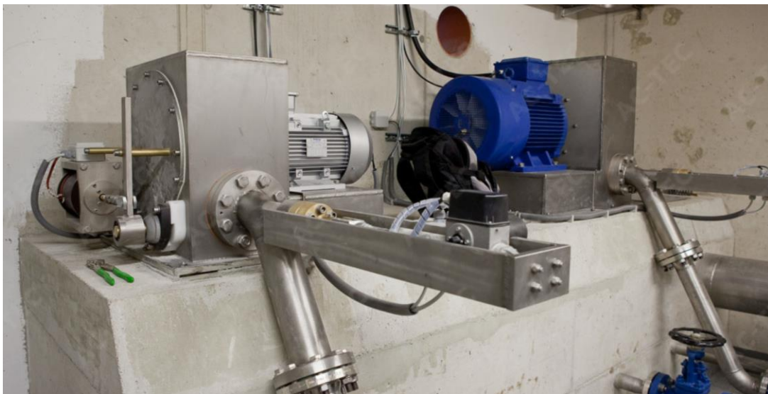
Figure E-21 Both turbines placed on their final position (AC-TEC, 2015)
