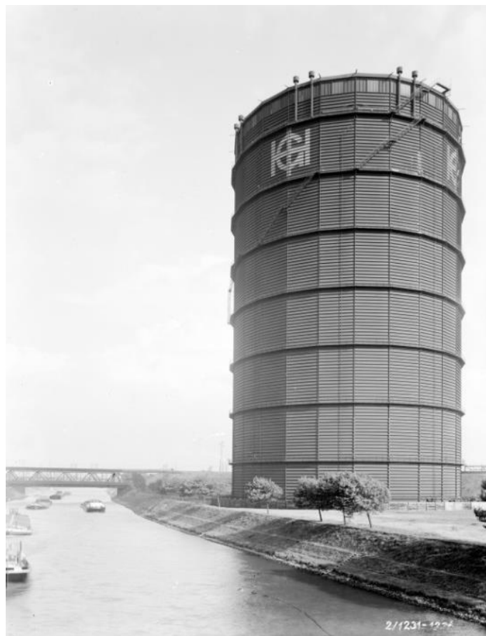
Figure A-13 The Gasometer in 1929, showing the logo of the Gutehoffnungshütte (Gasometer, 2016)
