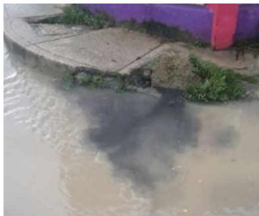
Figure 2.33: Sewage water leaking into the street after mild rainfall (Rafael Nuñez sector of Olaya)
