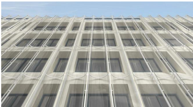
Image 97 - Cold bent glass in the façade. Image: Carlym Simoen.
