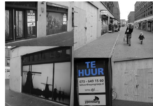
Figure 1.3: Vacant stores in Shopping Centre Ypenburg
