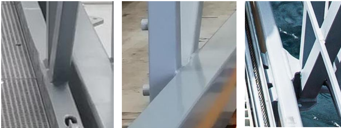
Figure 2. Eccentric joints used in Ampelmann's gangway systems.
