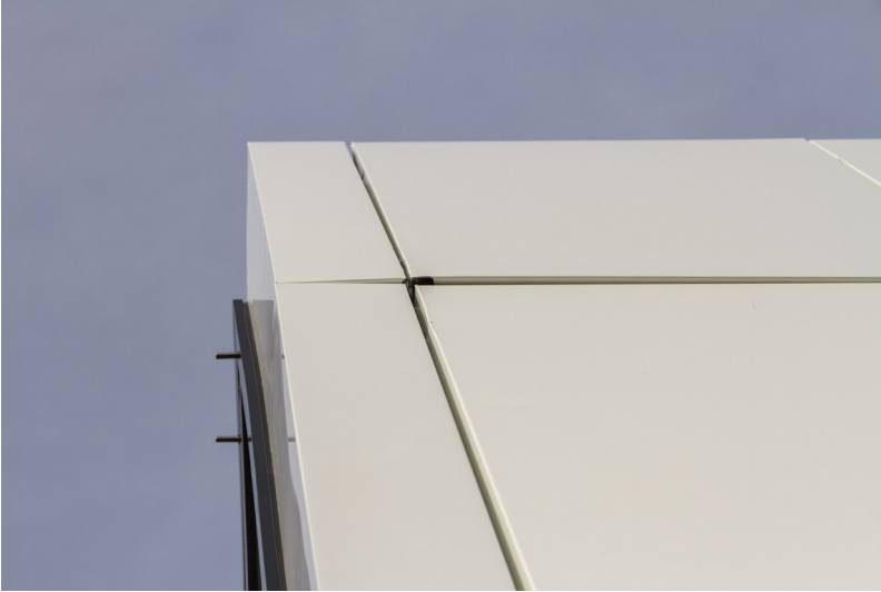
fig. 18. A lack of space for adjustment, causing unequal seams between cladding panels at the roof top (Bilow, 2017)
