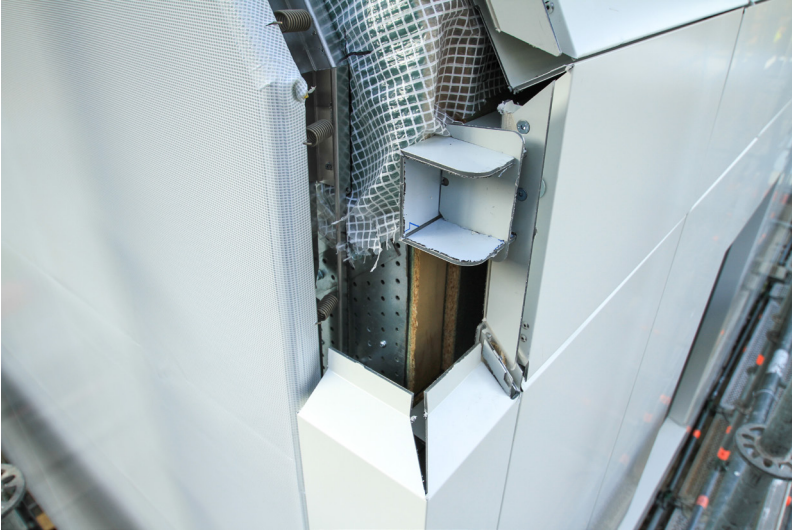
fig. 19. Gaps between the panel joints and surfaces (Bilow, 2017)
