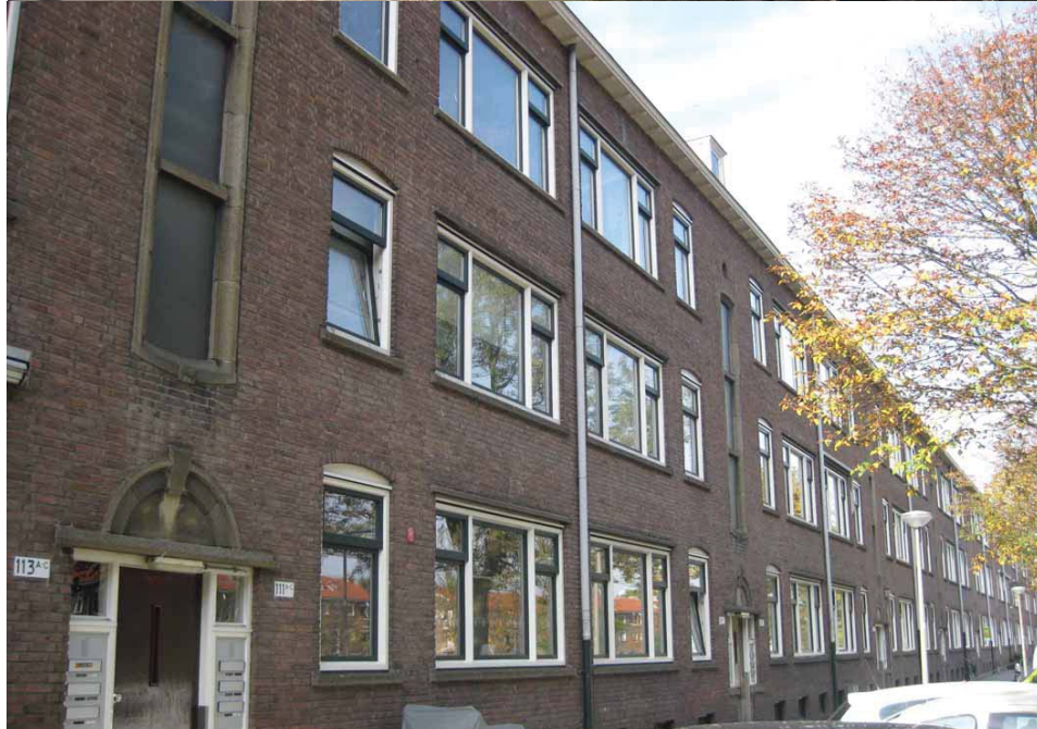
Fig. 81 (top) and 82 (bottom): Photo by the author. Though the monthly contributions of one is almost twice that of the other (top around €90 bottom €47) both have similar new window frames, new mailboxes and buzzer, and clean looking facade. Possible reason for this discrepancy is large repair or improved insulation, but
