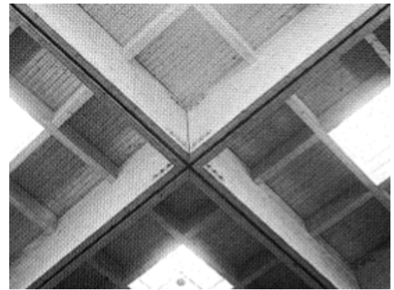
Figure3.4.17 Rigid (fixed) joint (Natterer,2004)
