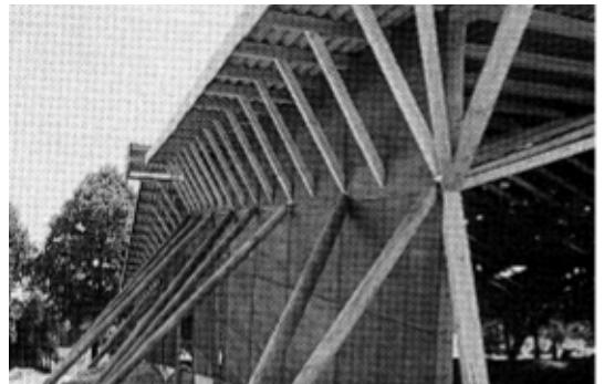
Figure3.4.13 Propped column (Natterer,2004)
