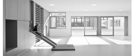
Figure3.4.22 New Kindergarten (Hurnaus,2011)
