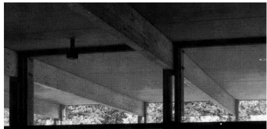
Figure3.4.12 Battened column (Natterer,2004)
