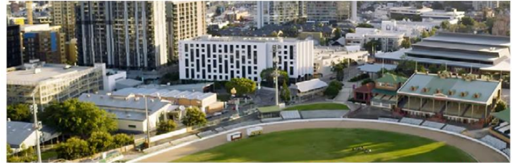
Brisbane Showgrounds Redevelopment. Lendlease + RNA
