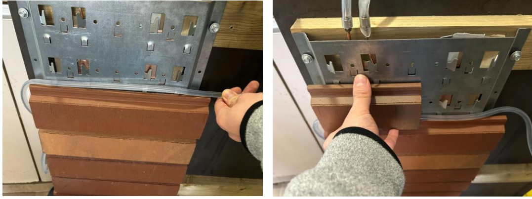
Figure 38: Solar collector water pipe installation. By author
