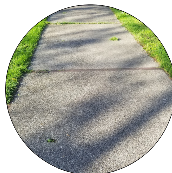
Figure 22. The concrete pavement
