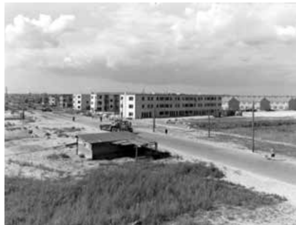
FIGURE 6 The Sloterveer Airey buildings shortly after construction, once slated for demolition are now being renovated.
