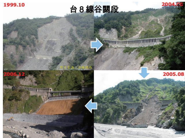
fig.17 The recurrent collapse and restoration of the Guguan section of Central Cross-island Highway.
