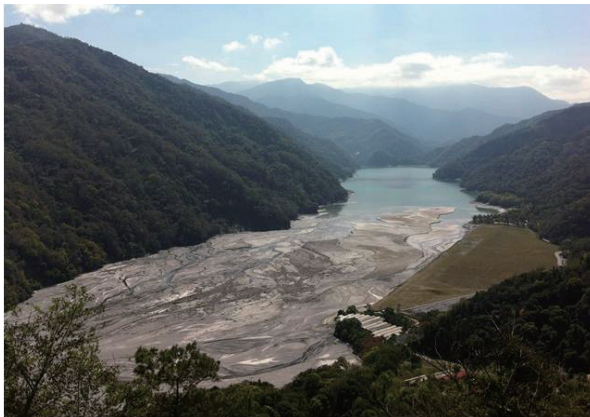
fig.11 Wushe (霧社) Reservoir 65% filled with sediment Source: Taiwan Academy of Ecology epaper (2013) [Online] http://enews.url.com.tw/ [accessed 20. Feb. 2017]
