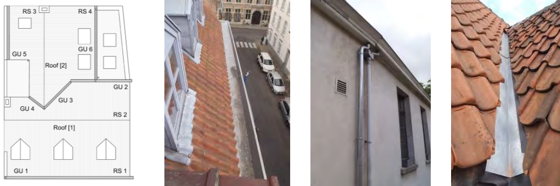
Figure 1: (1) Roof Plan, based on report Monumentenwacht, (2) Eaves gutter GU 1, (3) Eaves gutter GU 6, (4) Valley gutter GU 3, all pictures by Monumentenwacht
