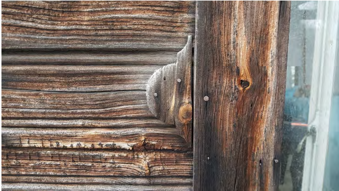
Figure 4: Decorative wooden pieces nailed on the cladding boards, 2017
