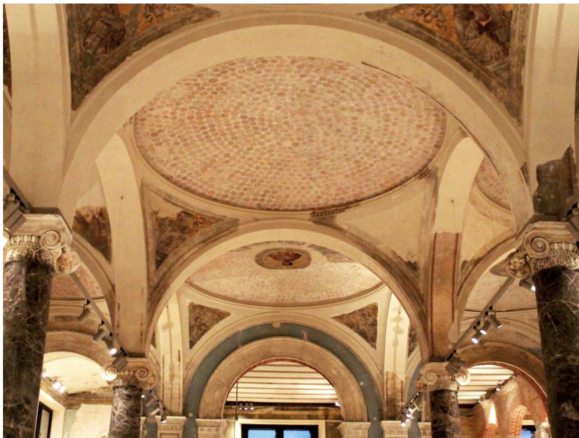
Figure 2: Germany, Berlin: the Neues Museum. Clay pots vaults designed by Friedrich August Stüler in the 19th century (L. Romano 2015).
