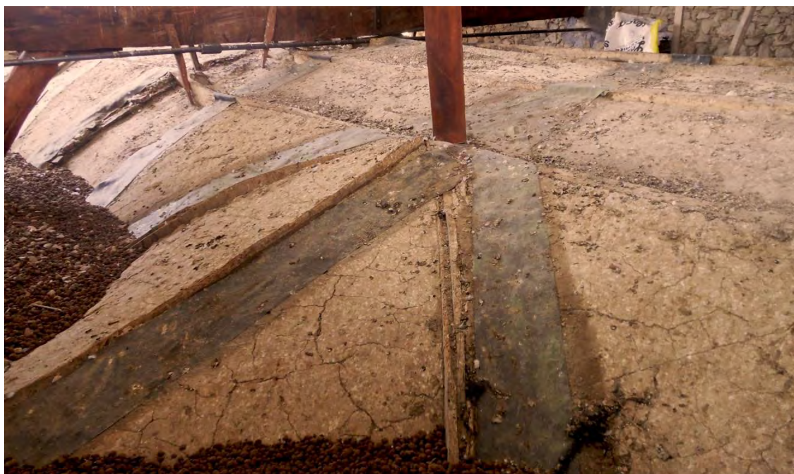
Figure 1: Italy, Baranello (Campobasso). St. Michele Arcangelo church. The extrados of the vault in the central nave: the image shows the wooden structure and the concrete made up of gypsum and lime (L. Romano 2016).
