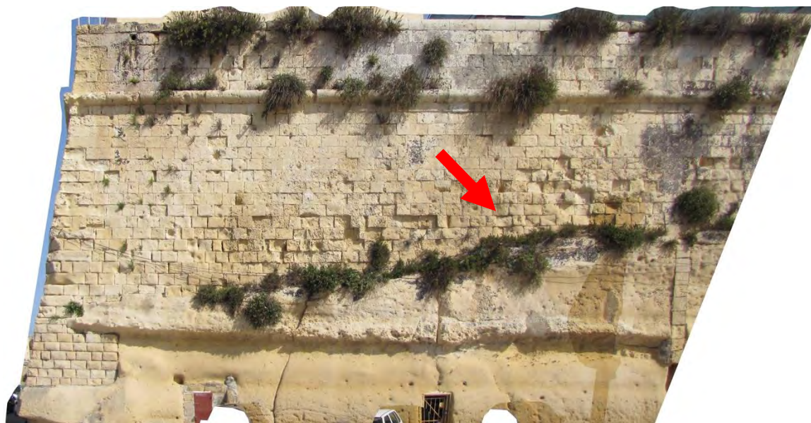
Figure 2: Rectified photography of Saint Sebastian Bastion, Valletta, showing area considered, (Restoration Directorate, Malta).
