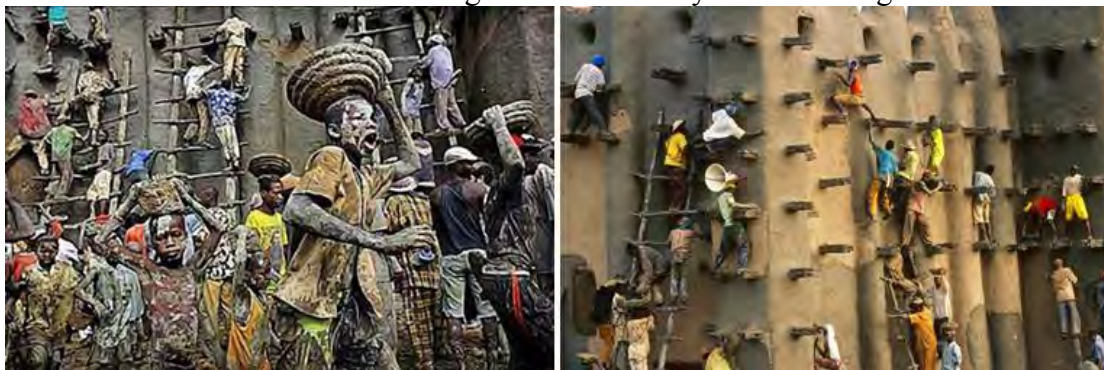
Figure 1-2: Crepissage de la Grande Mosquée (Plastering of the Great Mosque [3].
