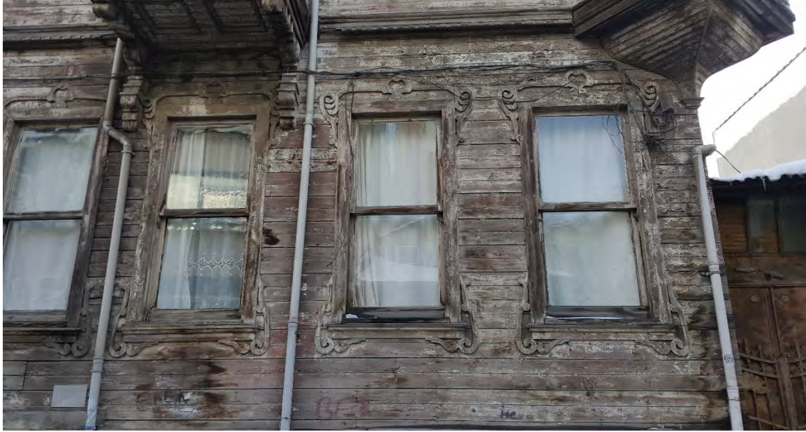
Figure 5: Guillotine windows and European style motives on the wooden cladding, 2016
