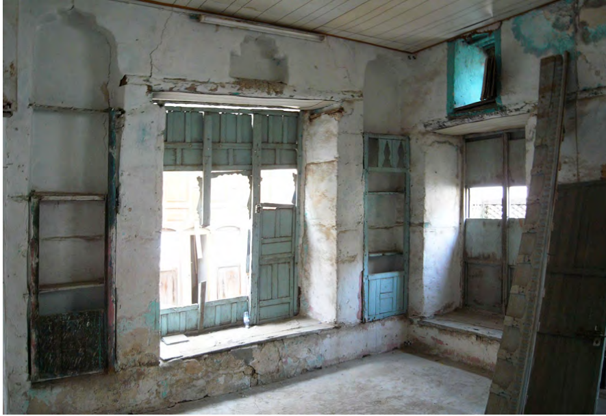
Figure 3: Condition of the Room 101 on the first floor of Al-Nawar House in the year 2011. The openings are facing in western and northern direction. The walls are constructed of load bearing coral stone blocks, covered with whitewashed lime plaster. The openings are filled with wooden shutters, which can regulate the airflow and daylight impact into the room [3].
