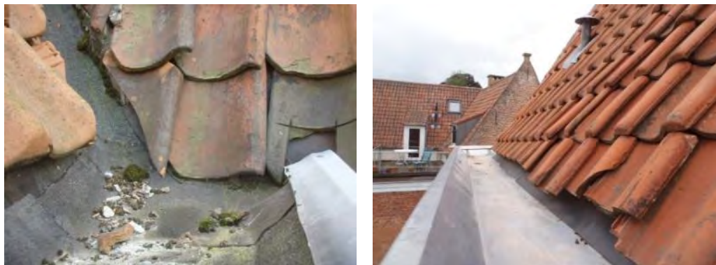
Figure 2: Left : gutters in asphalt, 2011. Right : new gutters in zinc, 2015. Pictures by Monumentenwacht
