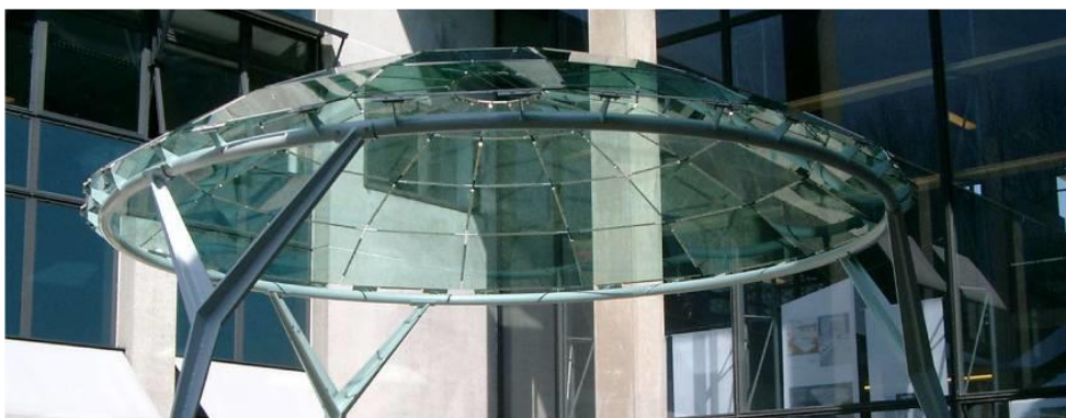
Figure 38: The all-glass dome outside of the former Bouwkunde building (Eekhout, Staaks, 2010)
