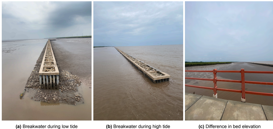
Figure 1.3: The current permeable breakwater, Pile-Rock Breakwater (PRBW), located in the study area at the coast of Bạc Liêu.
