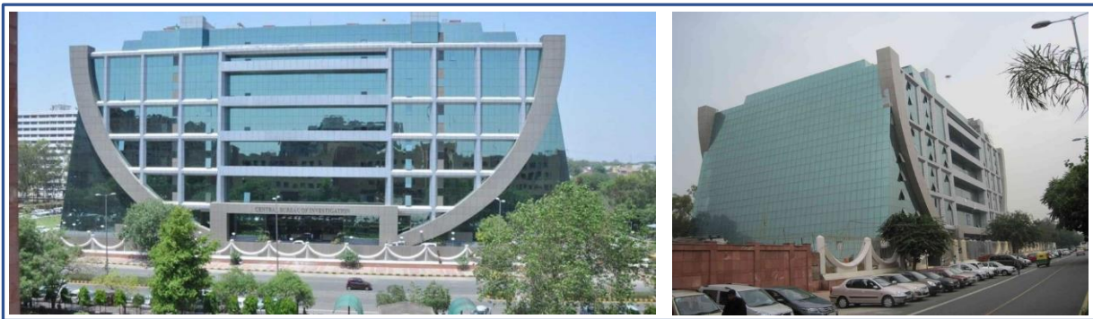
Figure 8.2: CBI Headquarters in New Delhi. A fully glazed façade using reflective glazing. A building design that has undergone criticism for its poor occupant comfort despite the use of reflective glazings and its high cost.
