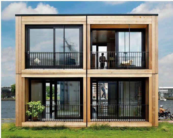
Figure 46 - Finch Buildings modular timber unit [51].
