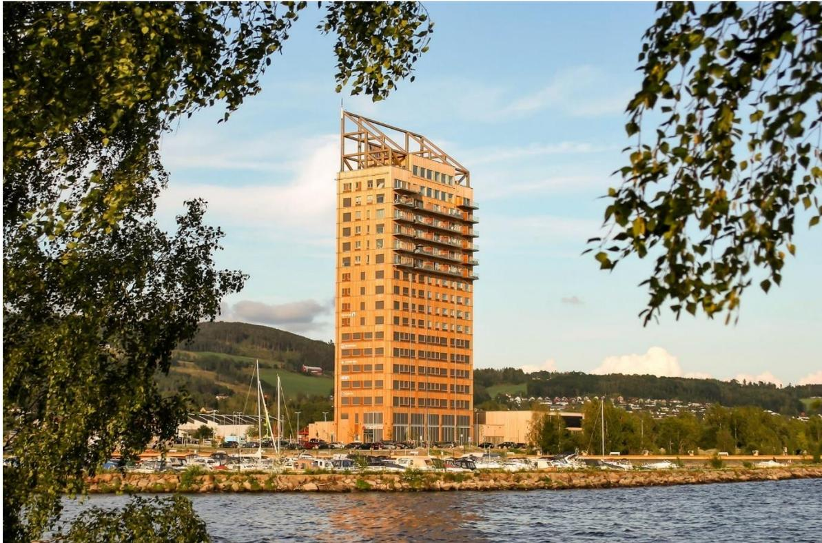
Figure 3 - The world's tallest timber building - Mjøstårnet in Brumunddal, Norway [7].
