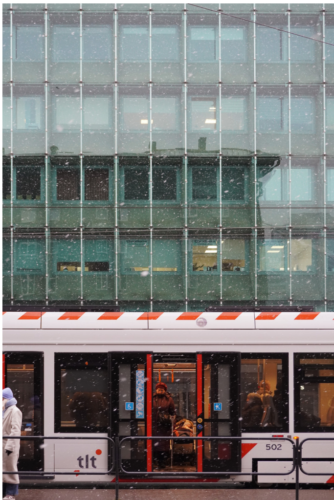
Soviet structure concealed by glass veneer (by author)
