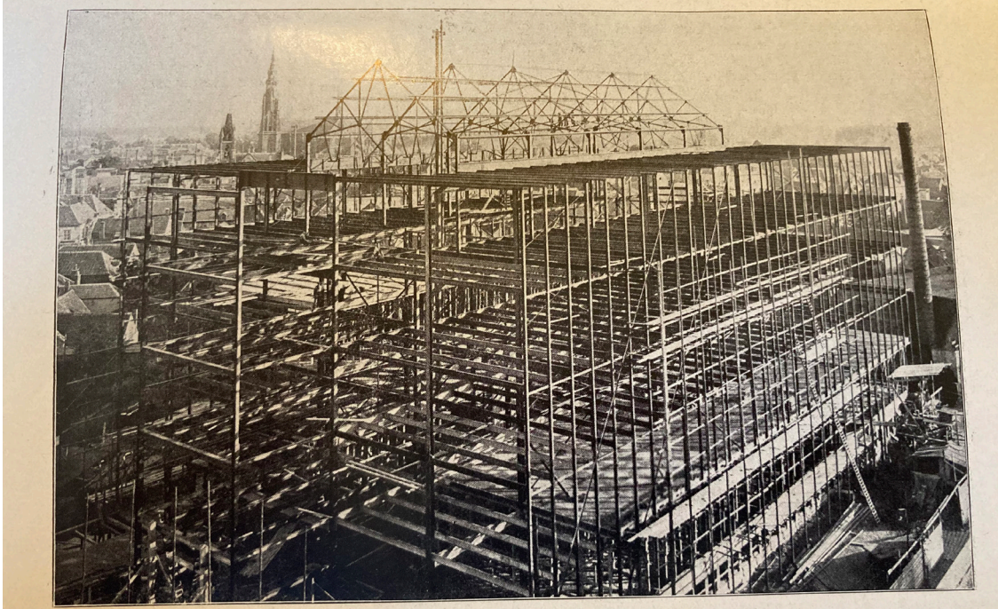
Figure 18. Construction of steel skeleton of the Bruine Heer. (Van Genderen. n.d.).
