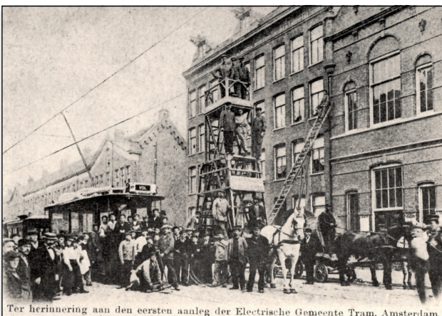
Image 3.4 Tensioning the overhead lines in the Marnixstraat on 2 August 1900 (Oxenaar, A., 1989, p. 88). The entire street observed how this innovative mode of transportation took shape.
