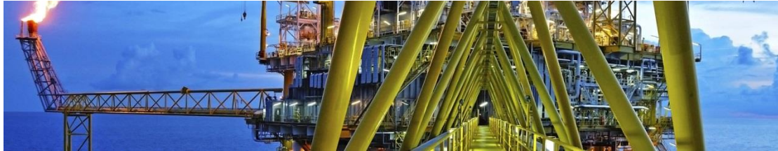
Figure 1. 1: Tubular steel members on offshore structures
