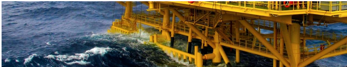
Figure 1. 2: Wave loading on tubulars members of support offshore structures
