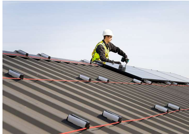
Figure I4: Pitched-roof (Sunbeam, n.d.)
