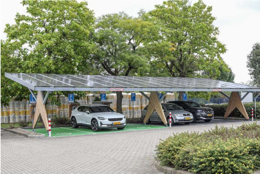
Figure 17: Carport with PV Panels (AmperaPark, 2024)
