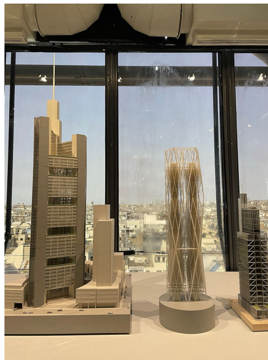
Fig. 1 Effect of condensation in the IGU cavity on the transparency of the glazing; Centre Pompidou, Paris
