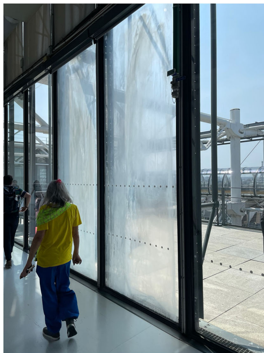
Fig. 1 Effect of condensation in the IGU cavity on the transparency of the glazing; Centre Pompidou, Paris
