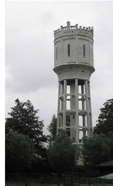
2. Early example of a reinforced concrete watertower
