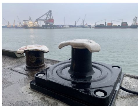
Figure E.1: Traditional bollard (left) and Smart Bollard (right) in the Port of Rotterdam (Rijnmond, 2021)
