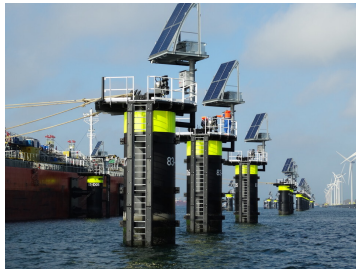
Figure 2.18: Mooring dolphins in the Port of Rotterdam (CROW, 2021)
