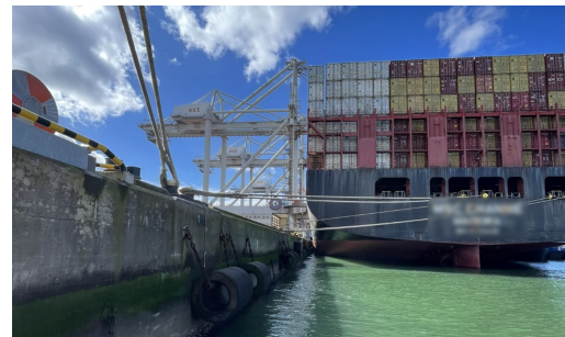
(b) DDN berth viewed from the landside
