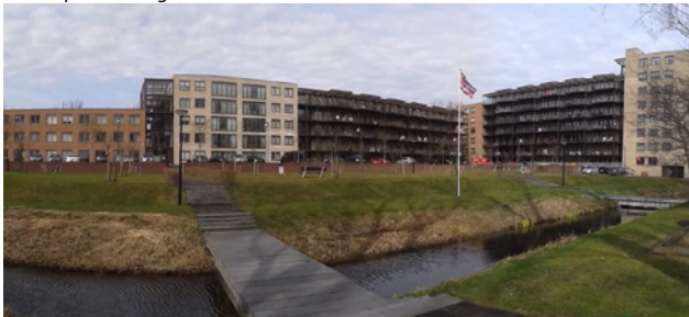
Semi-open building block in Alkmaar
