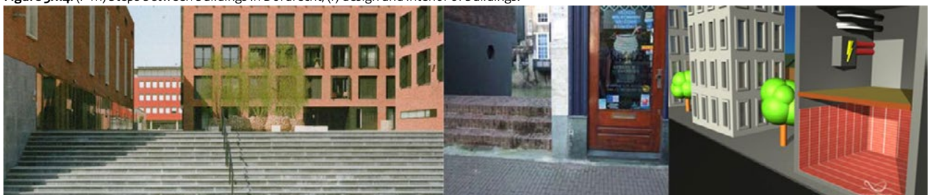
Figure 3.1.4: (l+m) Steps between buildings in Dordrecht; (r) design and interior of buildings.
