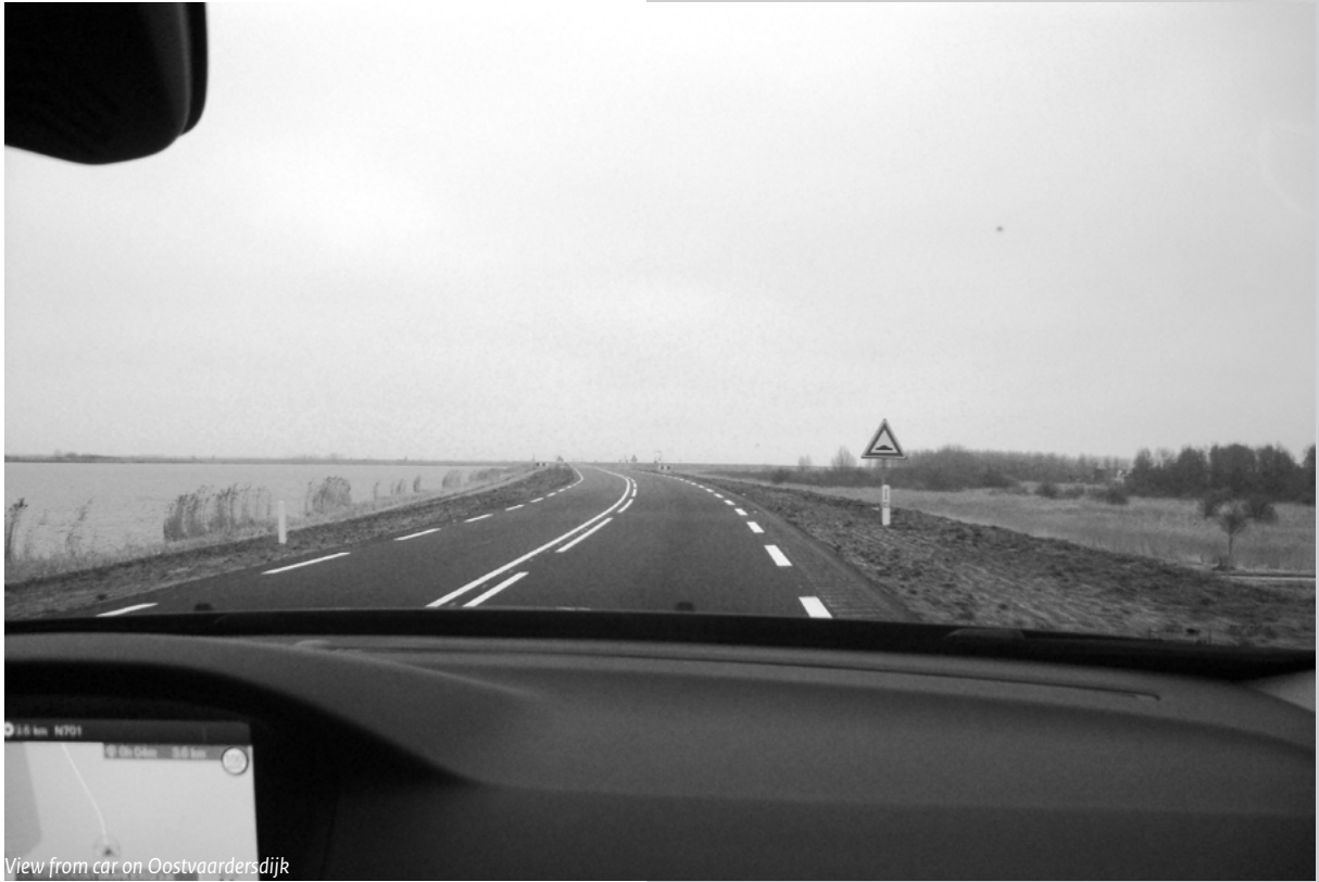
View from car on Oostvaardersdijk
