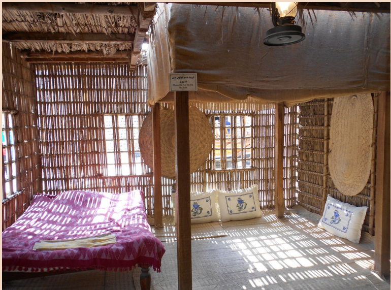
Figure 9, Arish (summer room) with open woven palm fronds for air flow (Where in Our World?, n.d.)
