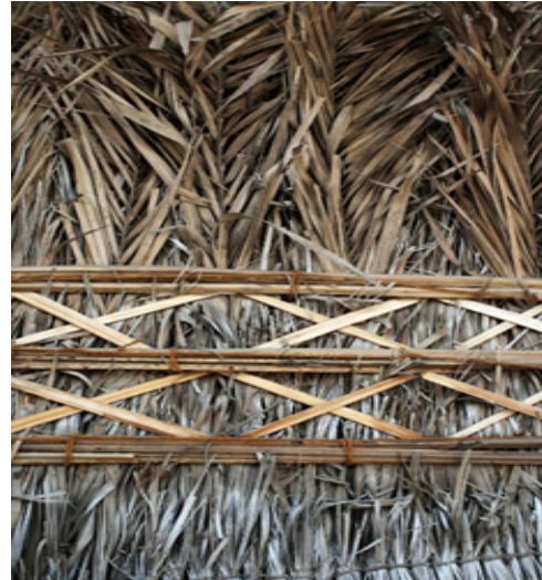
Figure 7, Arish wall constructed from palm fronds (The National, 2020)
