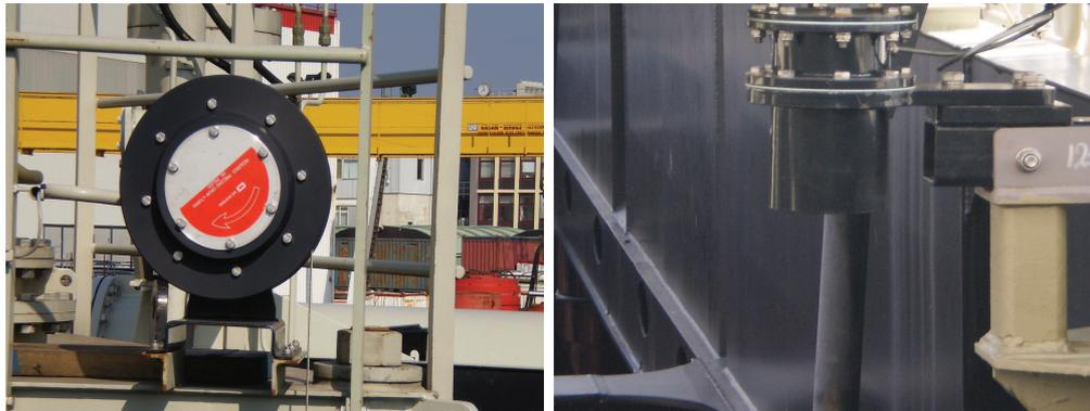
Figure 2.10: Sensors of the overflow height (left) and the mixture level (right).
