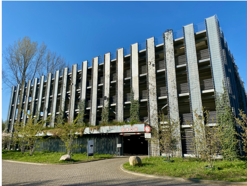
Figure 12.1: Parking garage P2 Sports at TU Delft.
