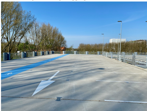
(c) The third quartile of the parking garage.
