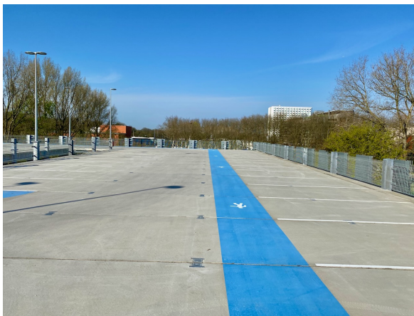
(a) The second quartile of the parking garage.
