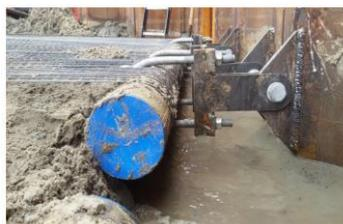
Figure 3: Connection of geogrid to SPW (Detert et al, 2019).
