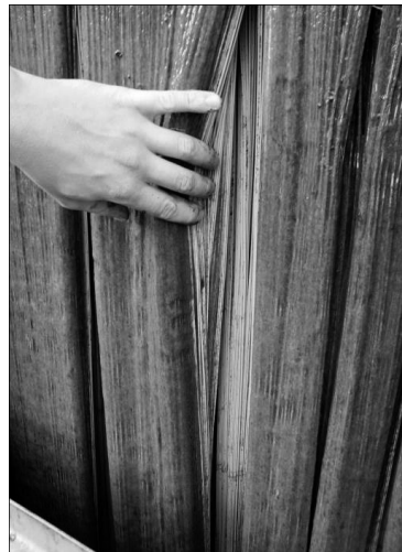
Figure 6.2: The effect of PVA wastewater on the membranes (picture Water Board Rijn and IJssel)
