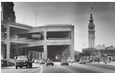
Fig.10: the Embarcadero Freeway. Gary Fong, The Chronicle, http://projects.sfchronicle.com/2016/sea-level-rise/part2/
