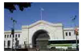
Pier 35 Bulkhead Building
