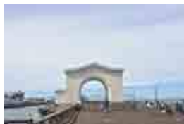
Pier 43 Ferry Arch
