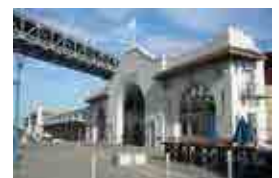
Pier 28 Bulkhead Building
