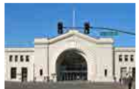
Pier 1 Bulkhead Building
